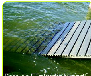
Roocycle ET plastic/wood post, bearers, joists, deck
