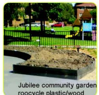
Roocycle ET raw x 50x200+100x200 "Cat Lyne" retaining wall 3 level curved
