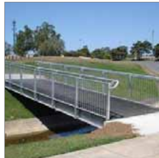
42430 Cycleway Bridge With Roocycle Decking
