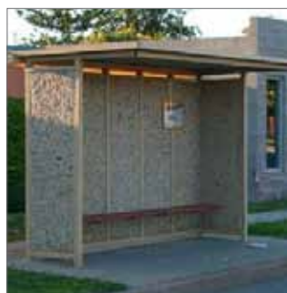
21944 Bus Shelter & Precast Panels Bush Hammer
