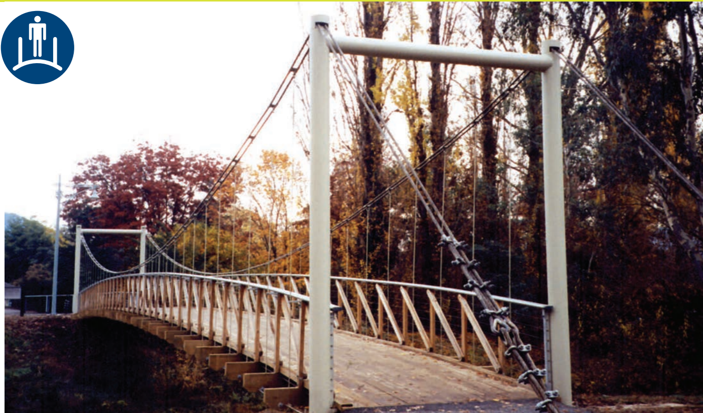
31735 35 m Span with 2.4 m Trafficable Width
