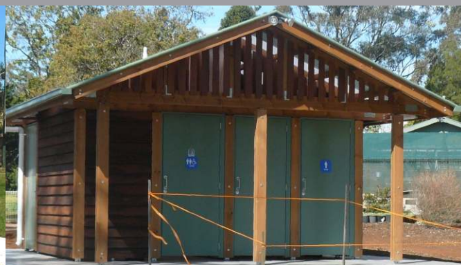
59806 Gordon - all timber, gable roof
