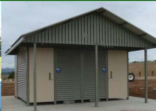
59801 Dalrymple - all steel, gable roof
