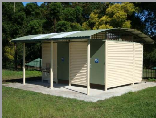
59885 Argyle - all steel, curved roof
