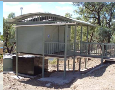
59880 Mackay - all steel, curved roof, alt waste
