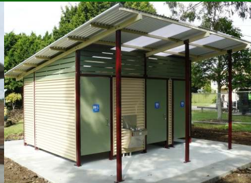
59812 Burley - all steel, skillion roof
