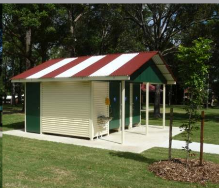
59802 Dalrymple - all steel, gable roof
