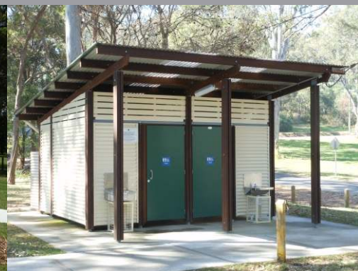
59816 Eyre - all timber, skillion roof
