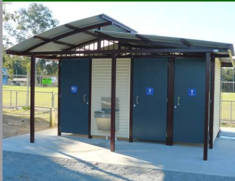
59795 Argyle - all steel, split roof
