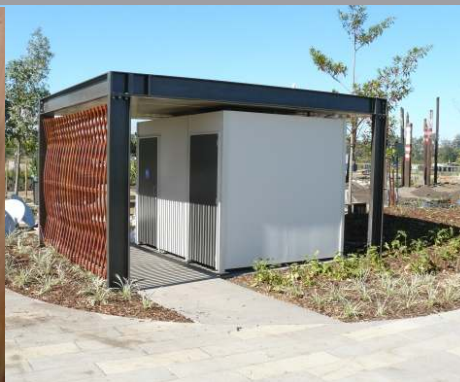
59790 Concordia Custom design restroom
