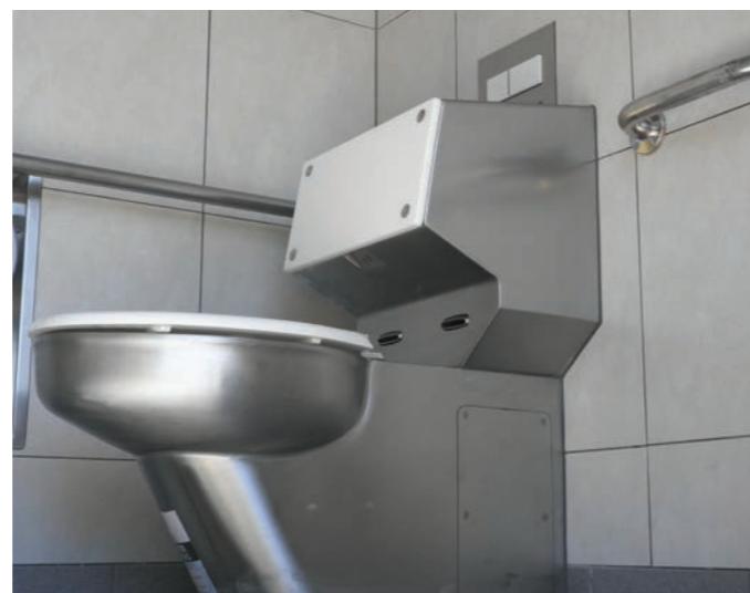
Toilet pan stainless steel. Note backrest and vents for air drying
